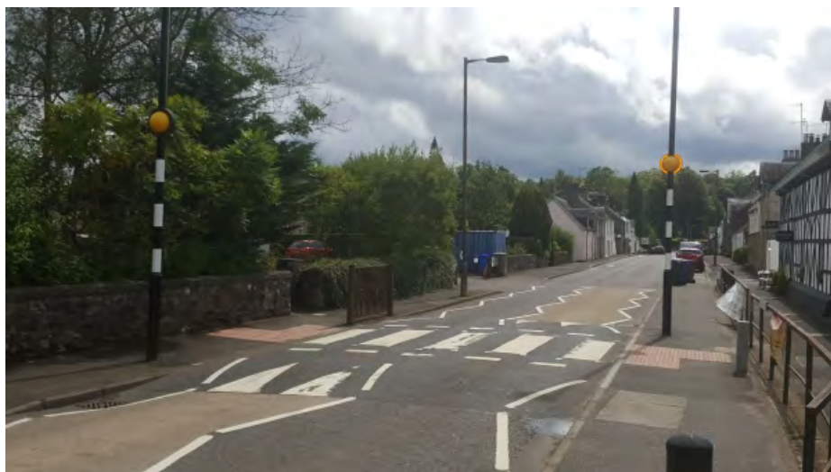
Raised platform with pedestrian crossing
